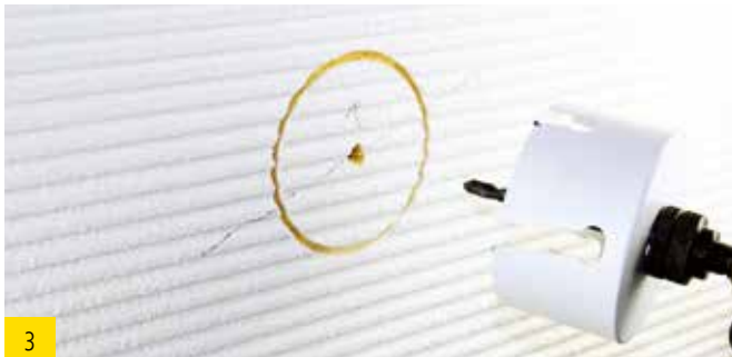
3 Pre-drilled plaster layer
