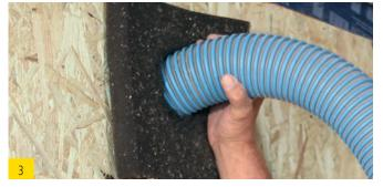
Inject air injected wood fiber insulation
