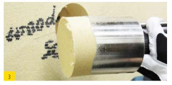
Remove drill hole plug
