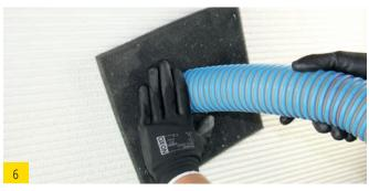
Inject air injected wood fiber insulation
