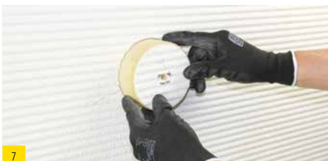
7 Insert drill hole plug ...
