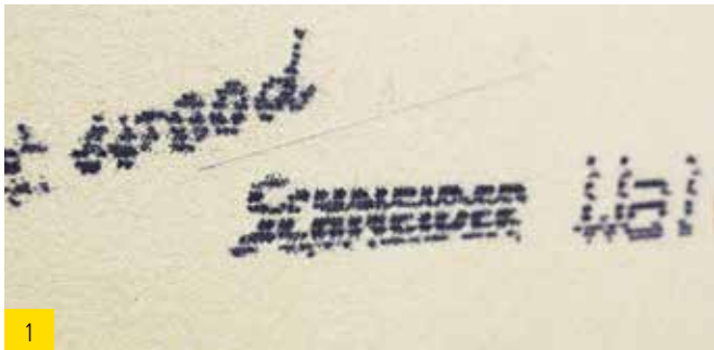
1 Mark and number the injection opening
