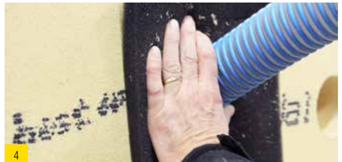
4 Inject air injected wood fiber insulation
