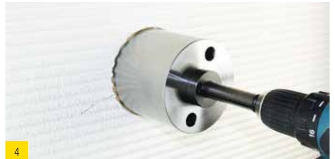
4 Make opening with keyhole saw (ED)
