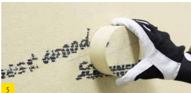
5 Insert drill hole plug ...
