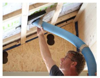
Fill roof structure using the hose procedure.
