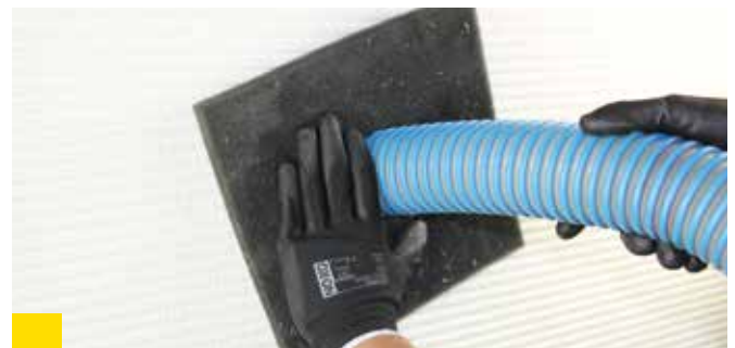
6 Inject air injected wood fiber insulation
