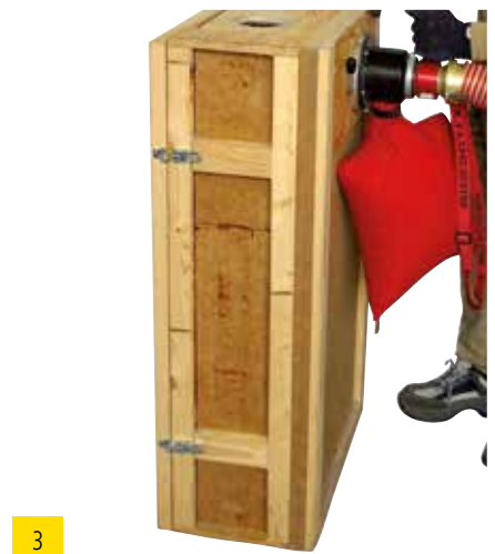
Compacted injection with ventilated rotary nozzle
