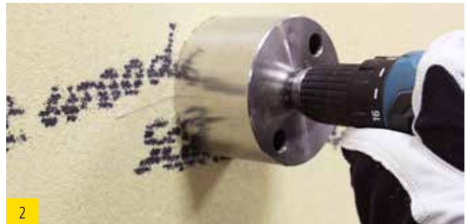
2 Make opening with keyhole saw (ED)
