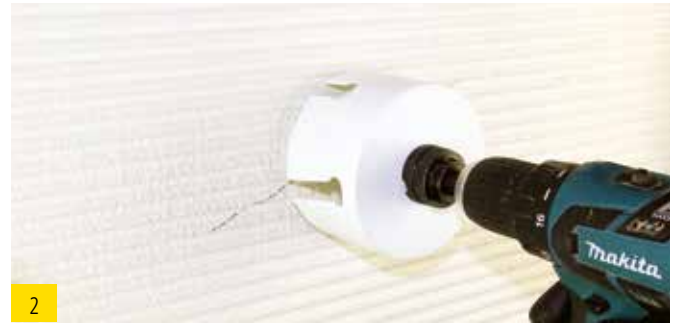
2 Pre-drill plaster layer with keyhole saw LH
