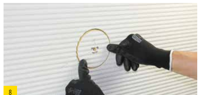
8 ... and push in flush with surface
