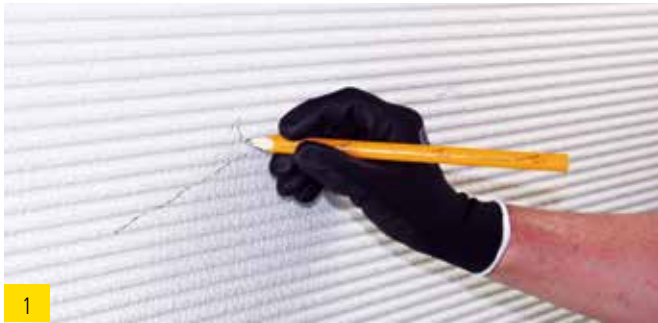
1 Mark and number the injection opening
