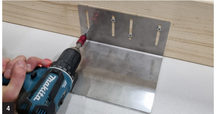
4 Screw bracket in waler. Remark: With board joints a bracket must also be provided in the vicinity of the joint.
