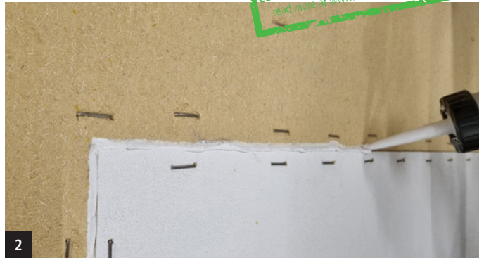
2 Fill the gaps in the facade level with FDM WALL
