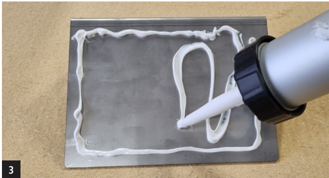
3 Apply FDM WALL to the bracket and press on to the back of the COVER PANEL FOR WINDOW LINTELS (see processing guideline for distances)
