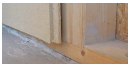
Cut off the groove side.
