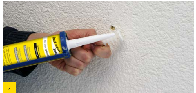
2 Application of best wood FDM WALL gap adhesive sealing compound for sealing purpose.
