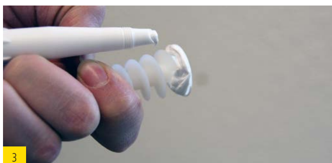
3 Application of best wood FDM WALL gap adhesive sealing compound under the anchor plate.
