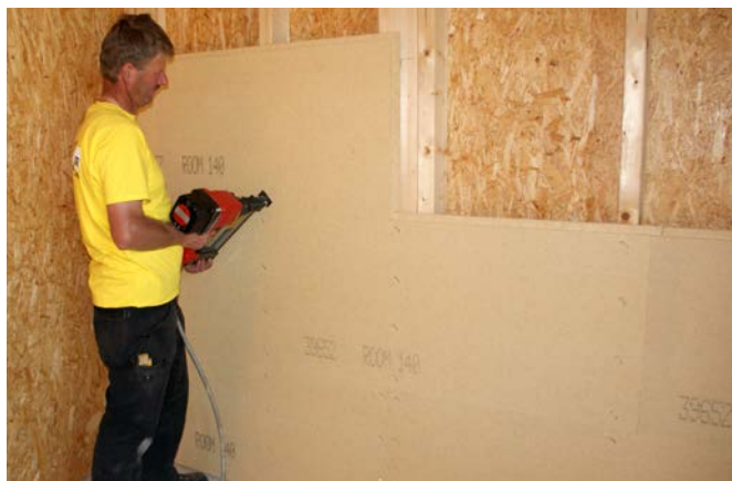
Fastening by means of broad back staples.
