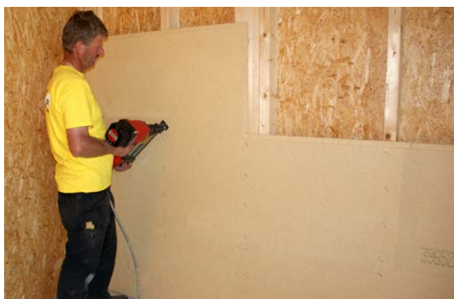
Fastening by means of broad back staples.
