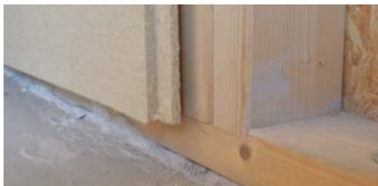
Cut off the groove side.
