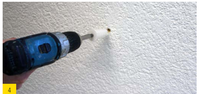
4 Flush insertion of the spiral anchor by means of a TORX T40 into the rendered wood fiber insulation board.
