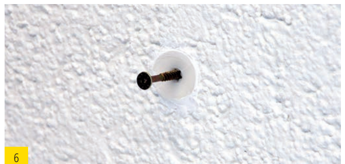
6 Fastening of the attachment piece by means of a 4–5 mm screw.
