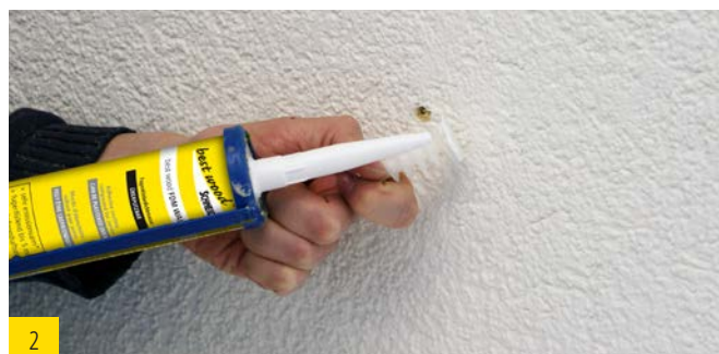
2 Application of best wood FDM WALLgap adhesive sealing compound for sealing purpose.
