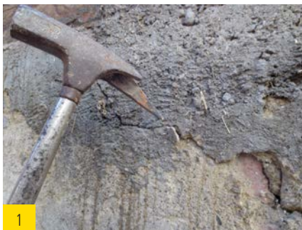
1 Remove all loose plaster.
