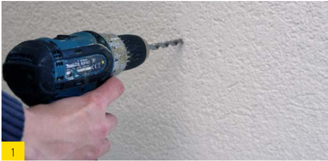
1 Pre-drilling of the rendered wood fiber insulation board by means of an 8 mm wood drill.
