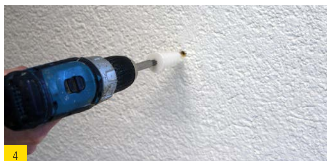
4 Flush insertion of the spiral anchor by means of a TORX T40 into the rendered wood fiber insulation board.
