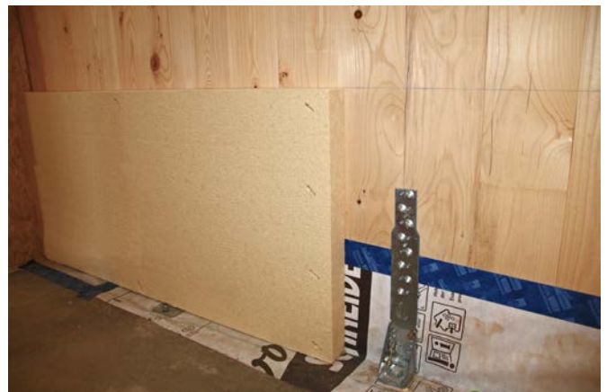
Horizontal alignment of the first row of panels by means of a marking chord.
