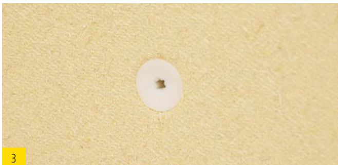
3 Flush-mounting of the spiral anchor.
