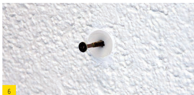
6 Fastening of the attachment piece by means of a 4–5 mm screw.
