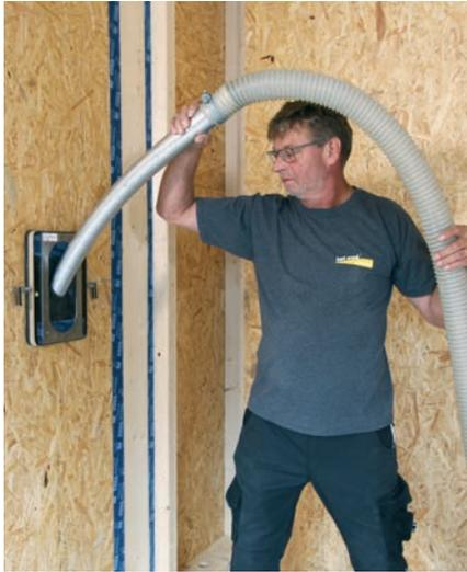
best wood FIBRE is installed using specially equipped injection machines. FIBRE is pumped in hoses under air pressure, fills the cavities of the various components and is compacted as per the instructions in this processing guideline. FIBRE may only be processed by trained and certified experts. This ensures that the air injected wood fiber insulation will be durable and long-lasting.
