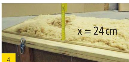
Determine the insulation thickness
