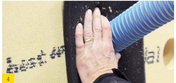
4 Inject air injected wood fiber insulation
