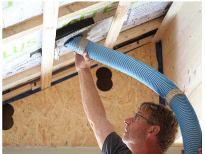
Fill roof structure using the hose procedure.
