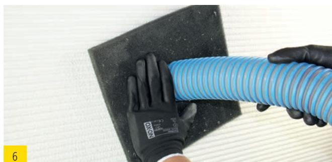
6 Inject air injected wood fiber insulation
