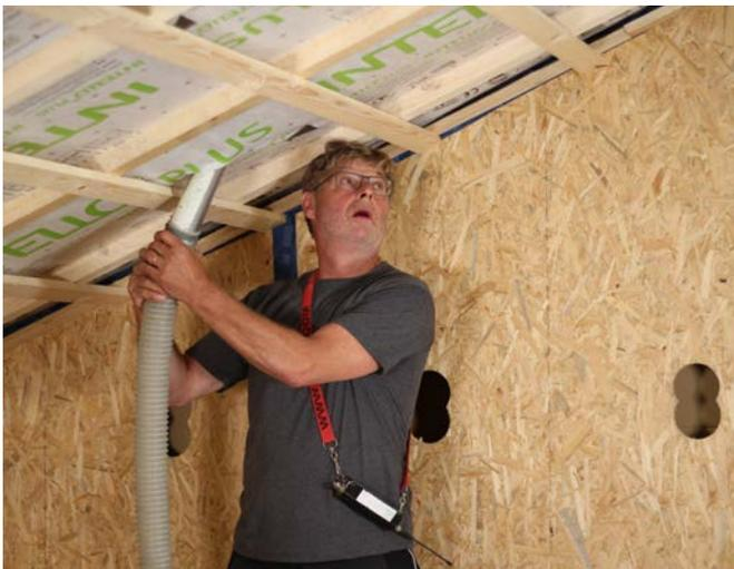
Fill roof structure with a 65 Ø needle.
