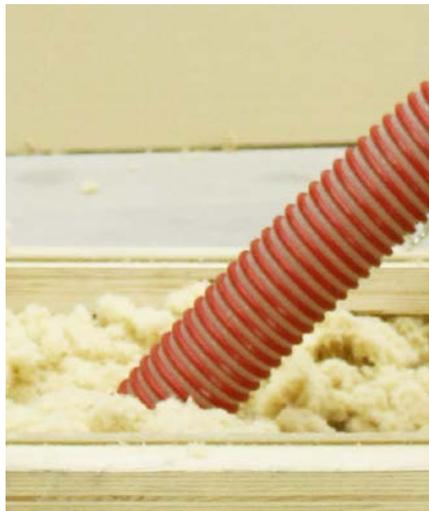
With the open blowing method, the insulating material is blown onto a surface that is open at the top. The top floor ceiling of a building is often insulated in this way. In the simplest case, application can be carried out using a hose or a rigid pipe.
