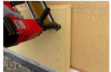
Fastening by means of stainless steel broad back staples.
