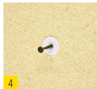
4 Fastening of the attachment piece by means of a 4–5mm screw.
