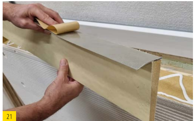
21 Pull off the adhesive tape from the sealing wedge which was cut to size previously
