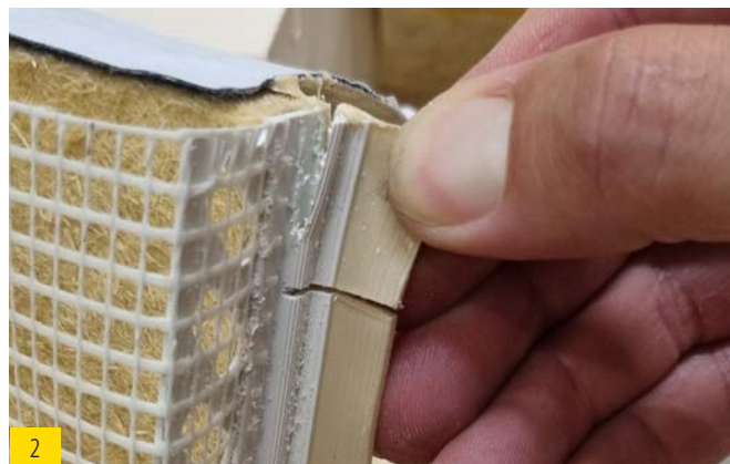
Shorten render stop bead including mesh web to marked length.
