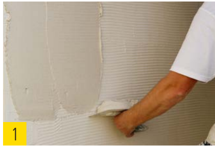
1 Application of vertical coating.
