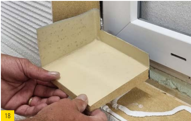
18 Position the sealing corners in both corners.
