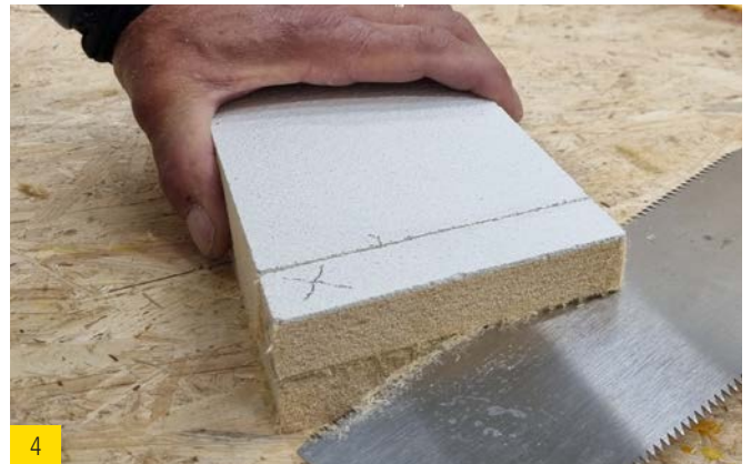
4 Saw out the marked area.
