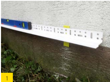
Base rail must be aligned and fastened horizontally.
