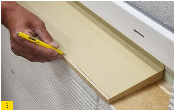
3 Mark sealing wedge with appropriate depth.
