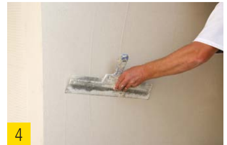
4 Embedding of the best wood reinforcement fabric.
