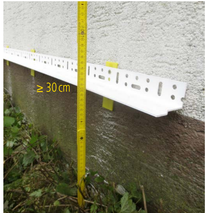
Splash water zone of \geq 30 cm without any additional measures.
