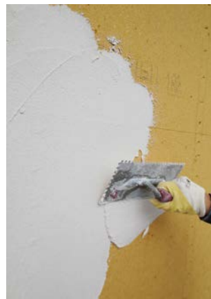
Application of adhesive and reinforcing mortar (UP).
