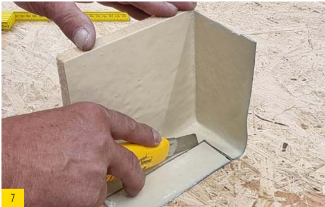
Adapt the sealing corners to the window corners.
