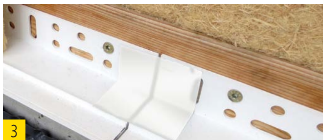
Bonding of the joint by means of an adhesive tape.
