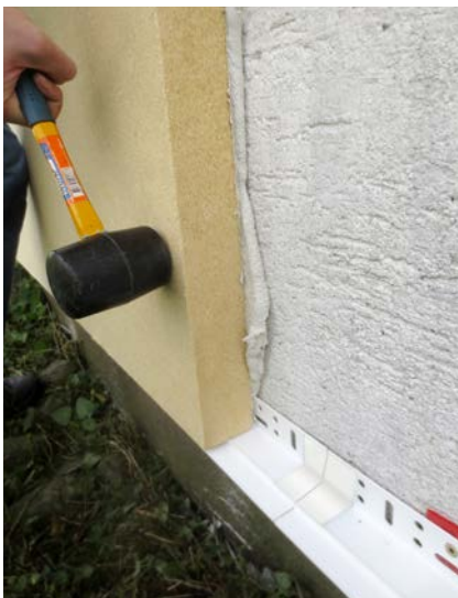
WALL 140 board has to be fitted fully into the base rail.
