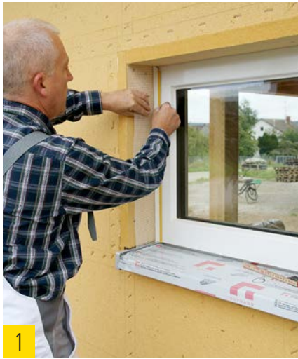
2 Architrave bead with telescope function sits flush to the inner edge of the window sill end piece.
