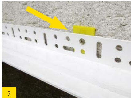
Distance adjustment at the base rail.
