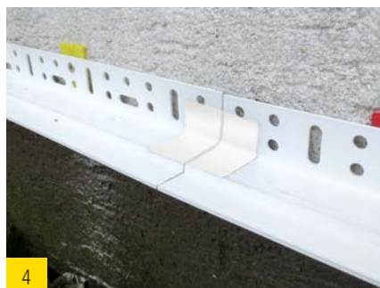
Bonding of the joint by means of an adhesive tape.
