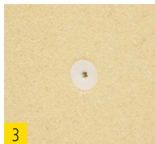
3 Flush-mounting of the spiral anchor.
