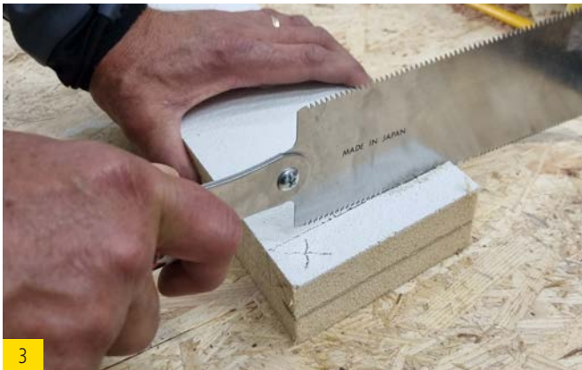
3 Cut out the marked area with a hand saw.
