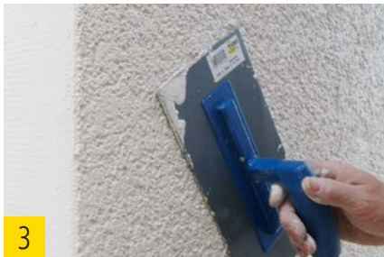
3 Structuring of the final render by means of a trowel.
