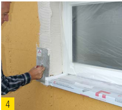
4 Application of adhesive and reinforcing mortar (UP) to the window reveal and the outer edge.
