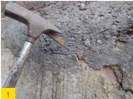
1 Remove all loose plaster.
