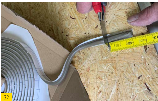
Cut off 4 cm of the sealing cord.
