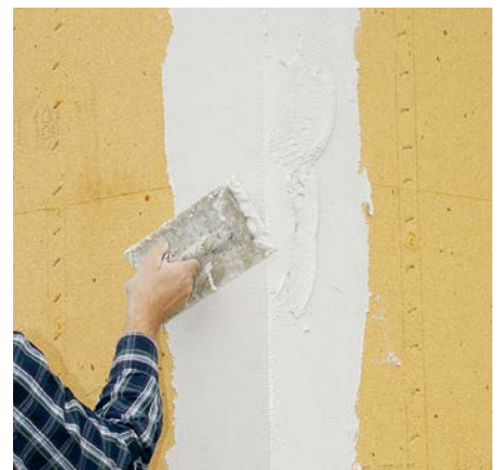
Embedding of the corner bead with fiber mesh.
