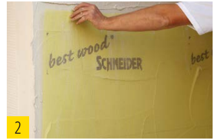
2 Application of best wood reinforcement fabric.
