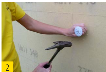
Application of the screw-in anchor.
