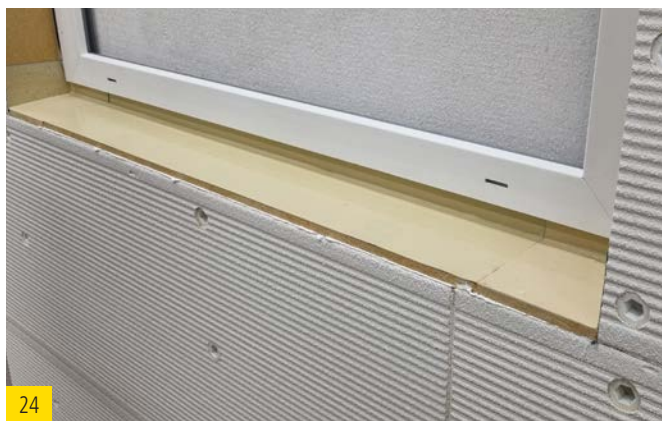
The ready glued and adapted sealing edge is now sealed at the butt joints and the render stop bead is fitted.
