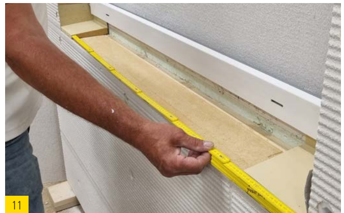
Measure the gap between the left and right sealing corners and shorten the sealing wedge (middle section) to the correct length.
