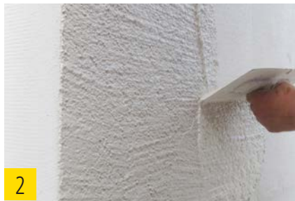
1 The final render is applied by means of a trowel and then skimmed to grain size.
