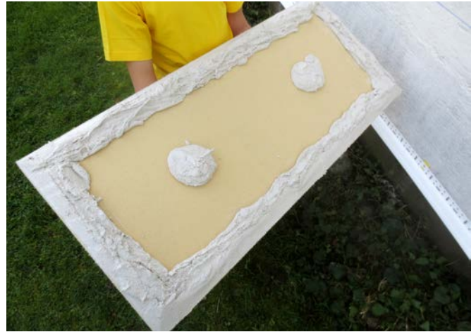
Application by means of the spot-and-bead method.
