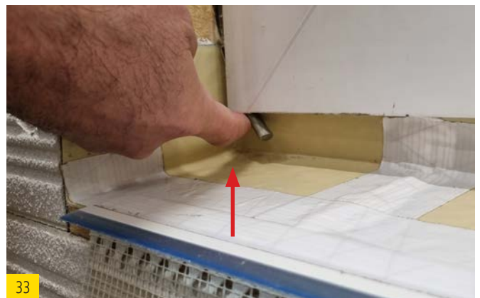
Affix the sealing cord in the corners beneath the window frame in the cavity so that it is closed.
