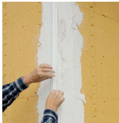
Application of corner bead with fiber mesh.
