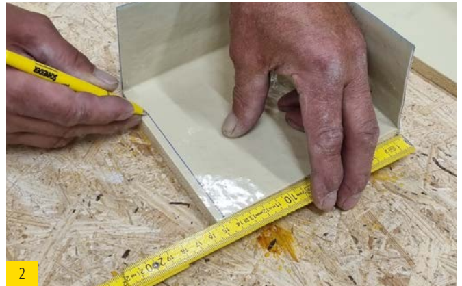
2 Mark sealing corner with appropriate depth.
