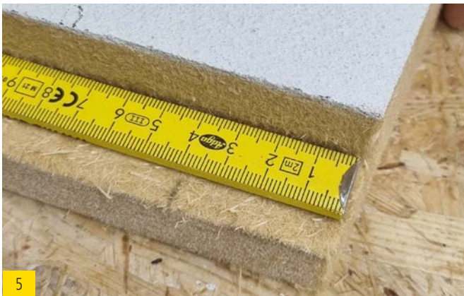
5 Measure 40 mm for notching the rear corner at the window.
