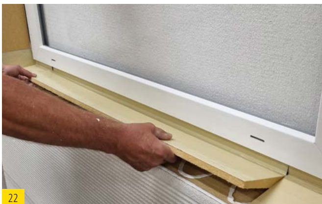
22 Push in the sealing wedge between the corners, fitting exactly
