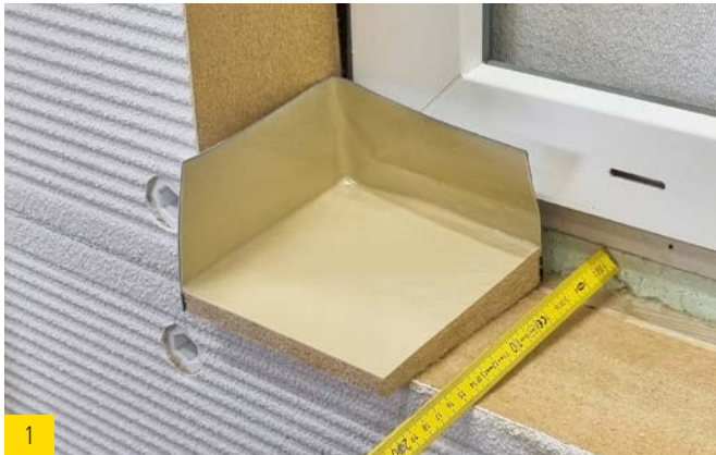
1 Measure depth of window sill.
