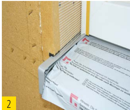
2 Architrave bead with telescope function sits flush to the inner edge of the window sill end piece.
