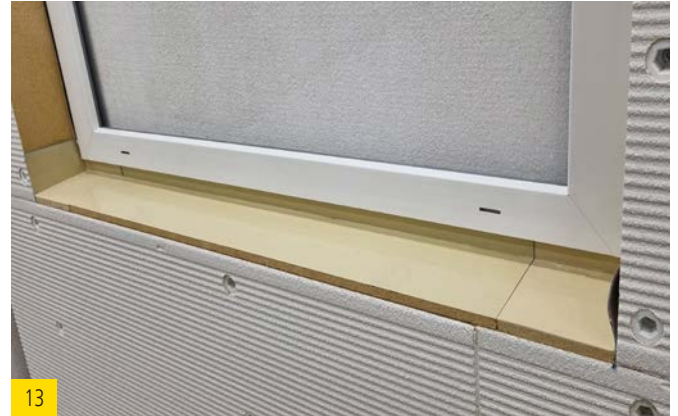
13 The front edge should be flush with the wall / wood fiber board. Remove all three parts again after checking.
