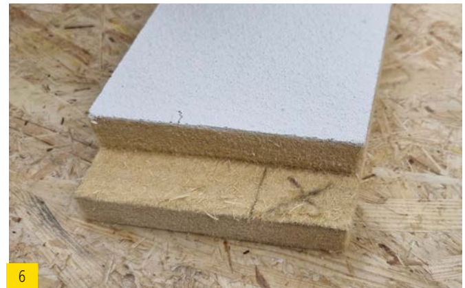
6 Saw out the marked area.
