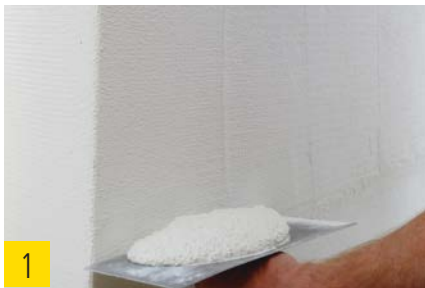
1 The final render is applied by means of a trowel and then skimmed to grain size.
