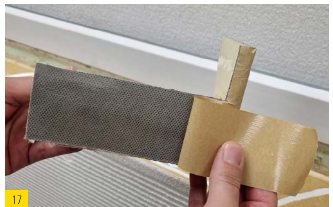
17 Remove the adhesive tape from the rear of the sealing corners.
