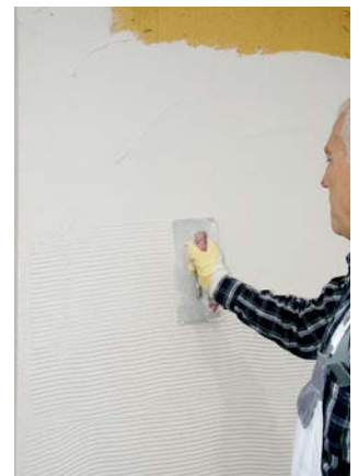
Application of serrated layer of mortar.
