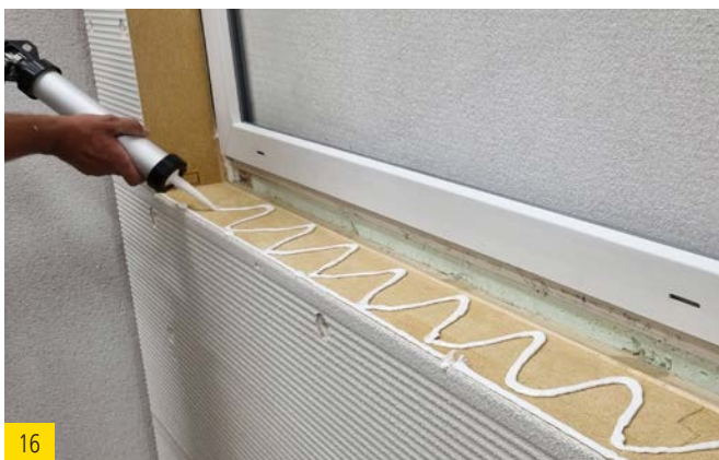
16 Apply a wavy line of best wood FDM WALL to the window sill.
