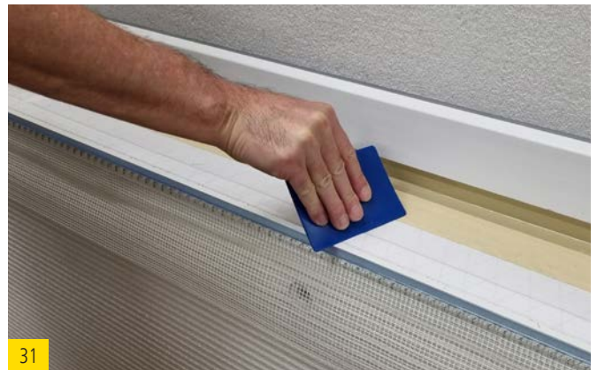
Smoothen the adhesive tape with a squeegee.
