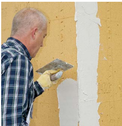
Application of adhesive and reinforcing mortar (UP).
