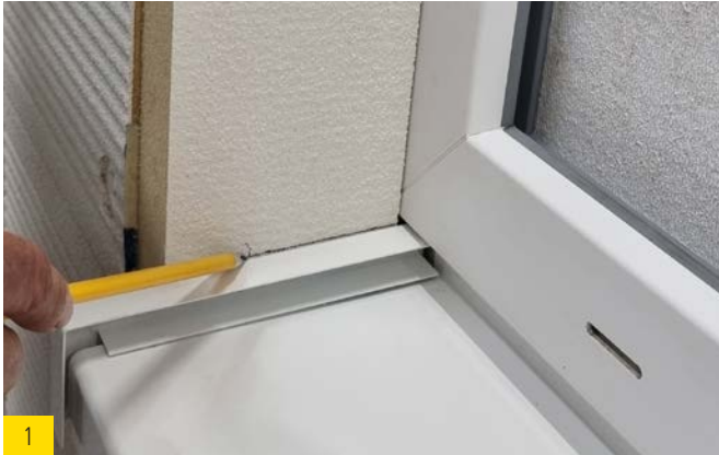
1 Notching of the 40 mm reveal board.
