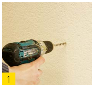
1 Pre-drilling of the unrendered wood fiber insulation board by means of an 8 mm wood drill.
