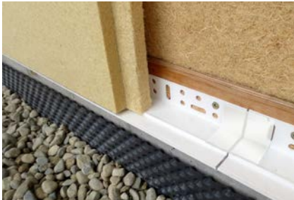
Cut off the groove side.
