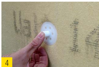
Application of the closing plug.
