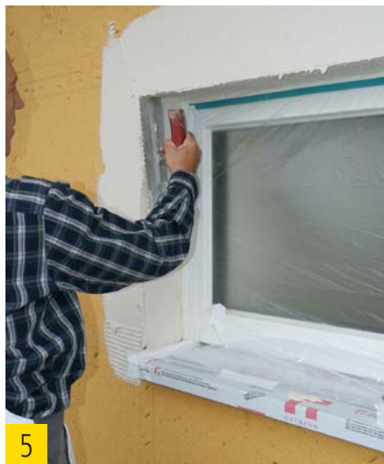
5 Embedding of the architrave bead with telescope function.
