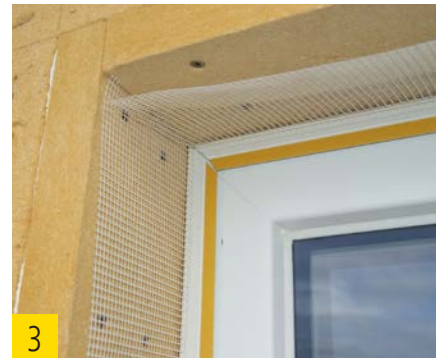
3 Architrave bead mitered in the edge.
