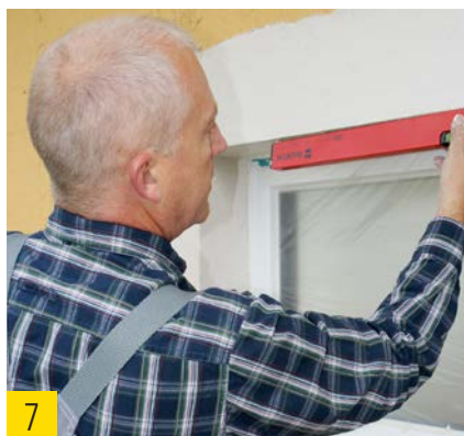
7 Horizontal and vertical alignment of the corner bead with fiber mesh.
