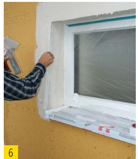
6 Application of corner bead with fiber mesh.
