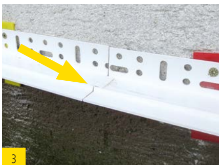
Installation of butt joint connectors at all longitudinal ends.
