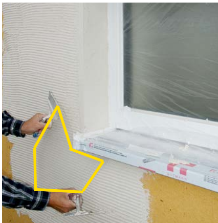
Embedding of reinforcing arrow.
