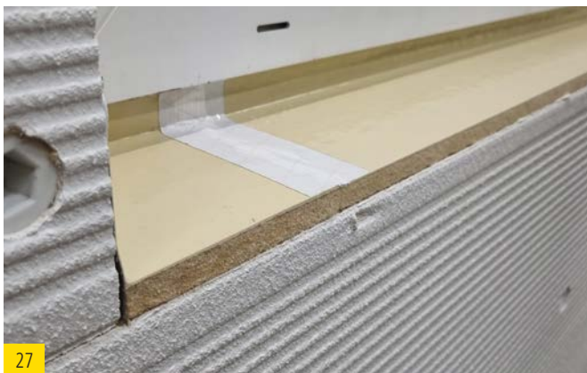
Firmly press down the TESCO VANA - use the same procedure at both joints.
