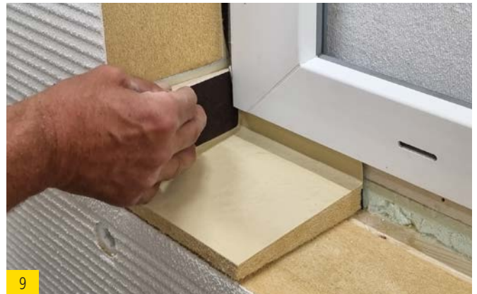
Insert both corner pieces and neatly press into the corner of the window sill using a tool (such as a wooden wedge).
