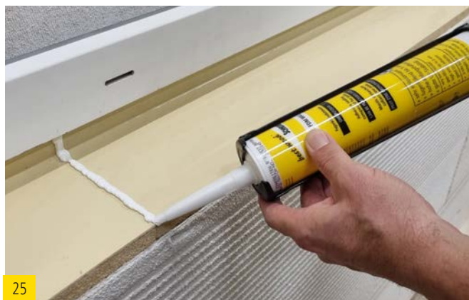
Seal the joint between the sealing corners and the sealing wedge with best wood FDM WALL.
