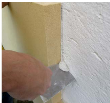
Remove any emerging adhesive.
