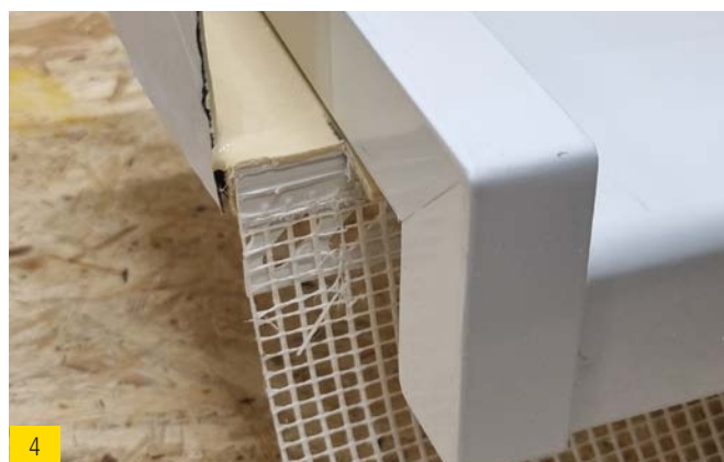
Render stop bead and window sill with same length.
