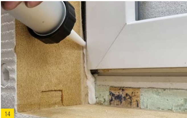
14 Fill the left and right corners with best wood FDM WALL.
