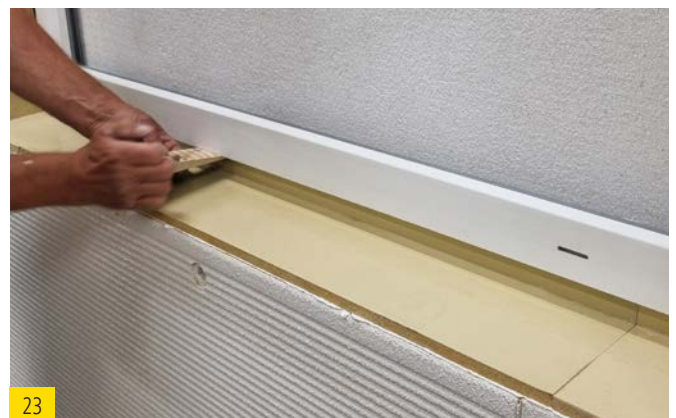
23 Also firmly press on the adhesive strip below the window frame using a tool (such as a wooden wedge)
