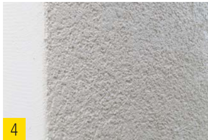
4 Ready structured plaster surface.
