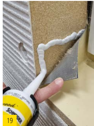
19 Apply best wood FDM WALL to the front. With the aid of a wedge, then press the sealing corner all the way in between the edge of the window and the wood fiber board.
