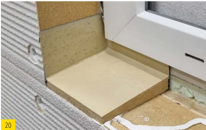
20 Important: Make sure that a "U" is formed again between the window frame and the wood fiber board (see picture no. 10)
