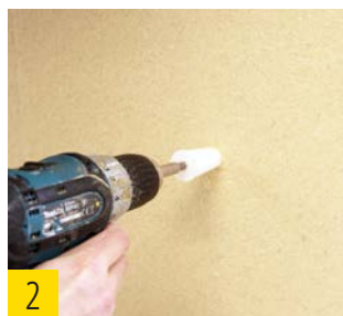
2 Insertion of the spiral anchor by means of a TORX T40 into the unrendered wood fiber insulation board.
