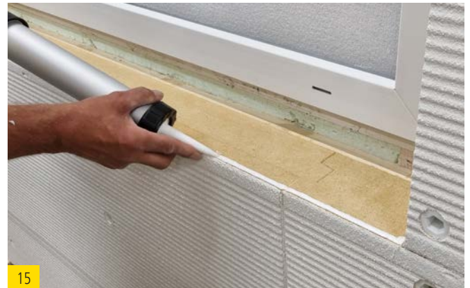
15 Apply best wood FDM WALL to the front edge.
