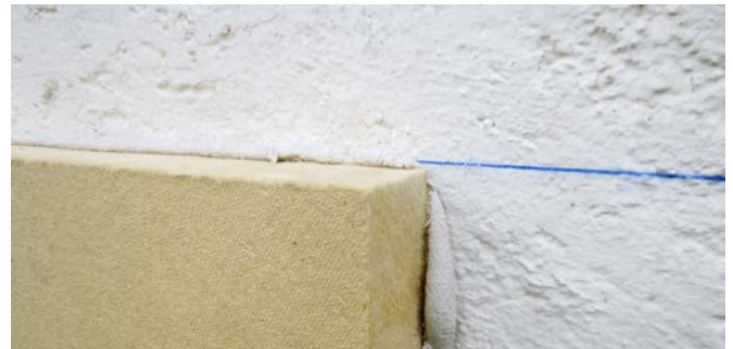
Horizontal alignment of WALL 140 boards by means of a marking chord.
