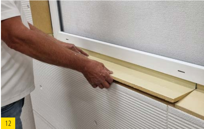
12 Push in the sealing wedge beneath the window frame and then check that the installation is correctly seated.
