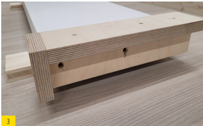
Place the installation aid on the bottom edge of the COVER PANEL FOR WINDOW LINTELS.
