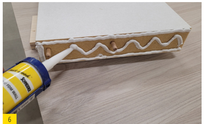
Apply FDM WALL to the front of an element and connect the elements together.
