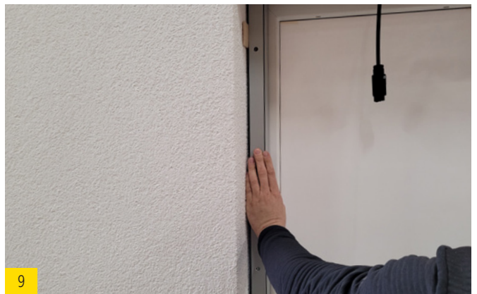
9 The distance to the render must be at least 5 mm.
