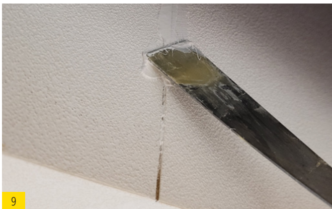
9 Open joints at the butt joint must be closed with FDM WALL.
