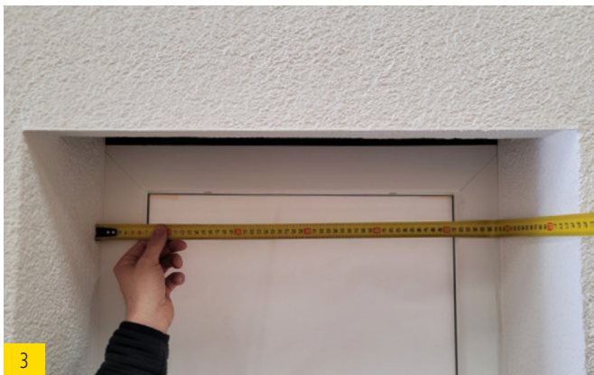
3 Check the width dimensions and, if necessary, mark on the total width of the sun protection
