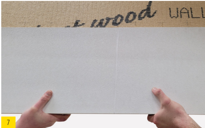
7 Lift the COVER PANEL FOR WINDOW LINTELS into the prepared opening with 2 people.
