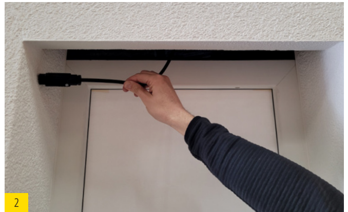
2 The cable is prepared and fitted with a Hirschmann connector. Cable length = 1/2 window width
