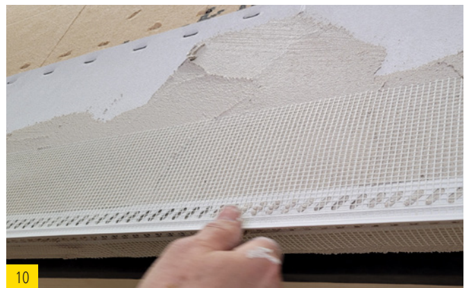
10 When embedding the drip edge profile, cut the fabric on the underside so that it does not protrude beyond the COVER PANEL FOR WINDOW LINTELS. The joint of the COVER PANEL FOR WINDOW LINTELS and the joint of the drip edge profile must be offset.
