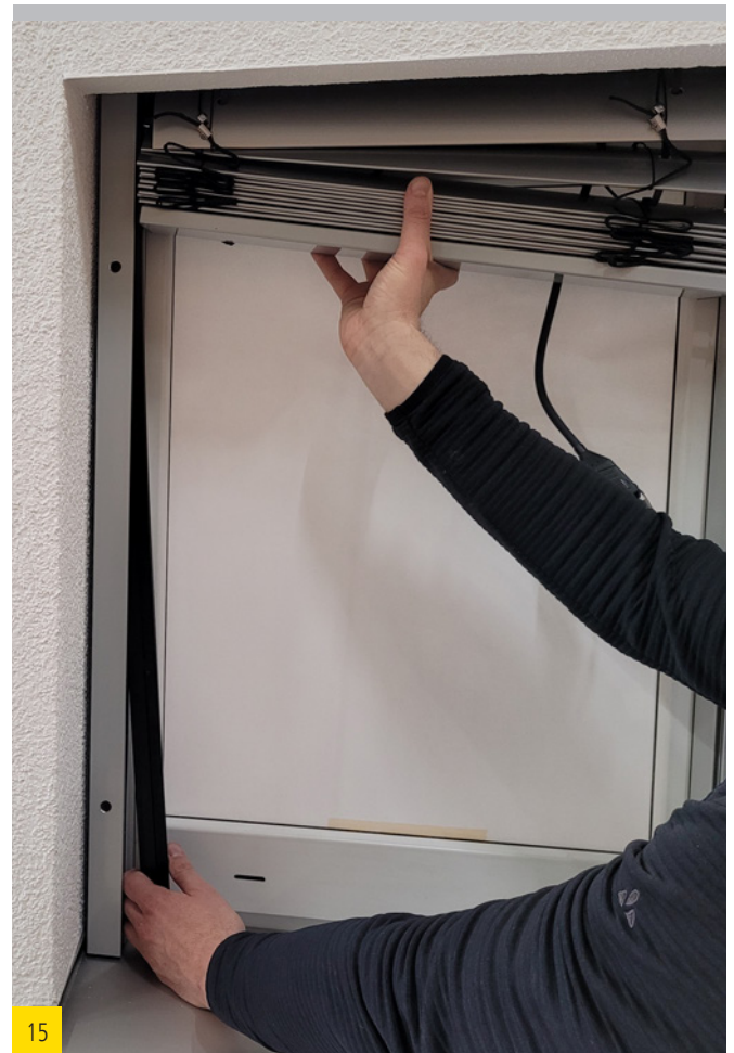
14 Align the outdoor blind along the width and slightly tighten the screws at the base.
