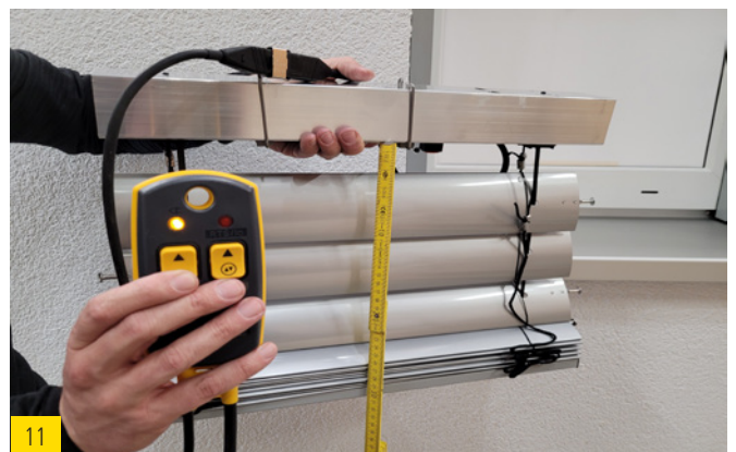
11 Connect the drive cable and lower the outdoor blind by approx. 20 – 30 cm.
