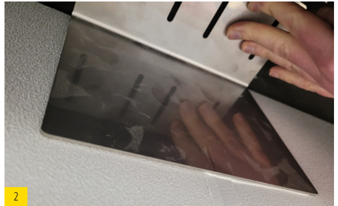
2 Press bracket onto rear of cover panel for window lintels
