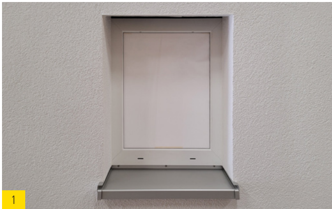
1 All rendering and painting work has been completed.
