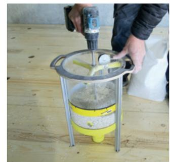
Put the chippings into the CLT BOX – CEILING FS using a cordless screwdriver **and low speed**.
