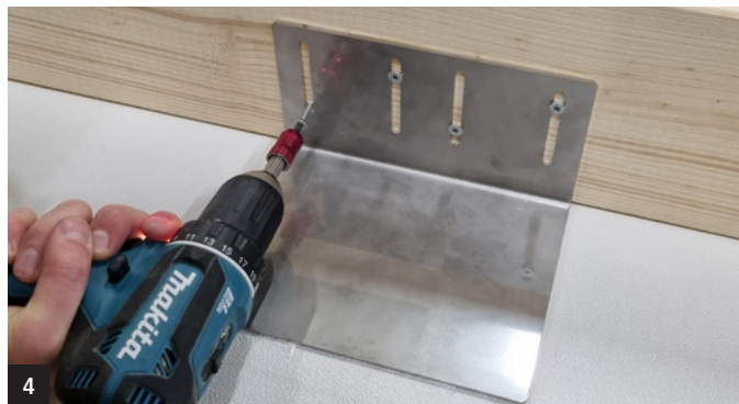
4 Screw bracket in waler. Remark: With board joints a bracket must also be provided in the vicinity of the joint.
