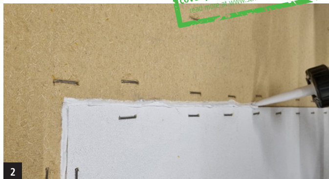
2 Fill the gaps in the facade level with FDM WALL
