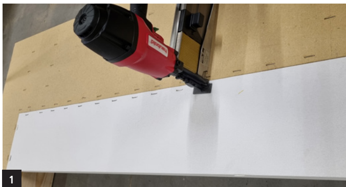
1 Staple COVER PANEL FOR WINDOW LINTELS all round at half the stanchion / waler width
