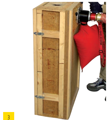
Compacted injection with ventilated rotary nozzle
