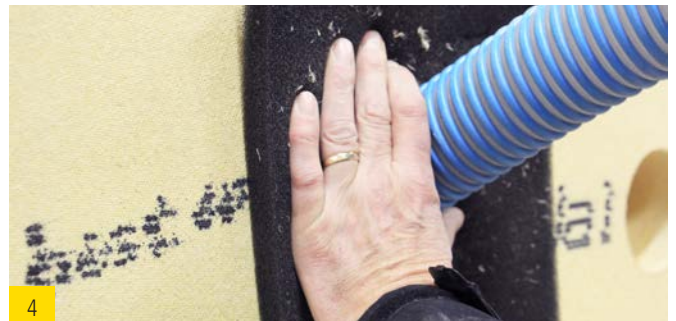
4 Inject air injected wood fiber insulation
