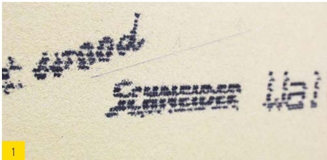
1 Mark and number the injection opening
