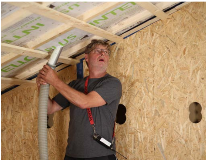
Fill roof structure with a 65 Ø needle.
