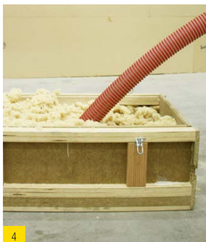
Open blowing with hose
