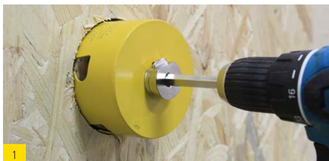
1 Make opening with keyhole saw LH
