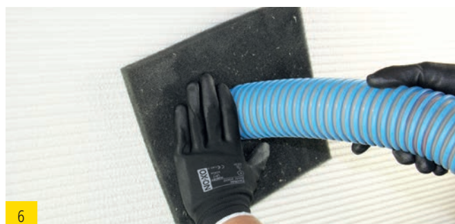
6 Inject air injected wood fiber insulation
