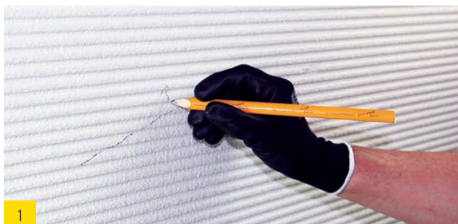
1 Mark and number the injection opening
