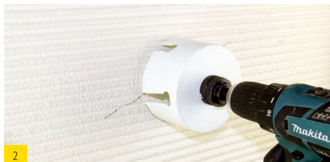
2 Pre-drill plaster layer with keyhole saw LH
