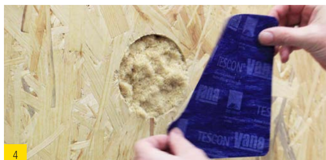
4 Close opening with adhesive patch
