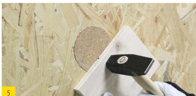
5 Close off with cork plug in the event of fire safety requirements
