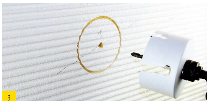
3 Pre-drilled plaster layer
