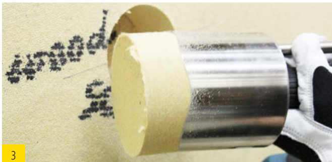
3 Remove drill hole plug
