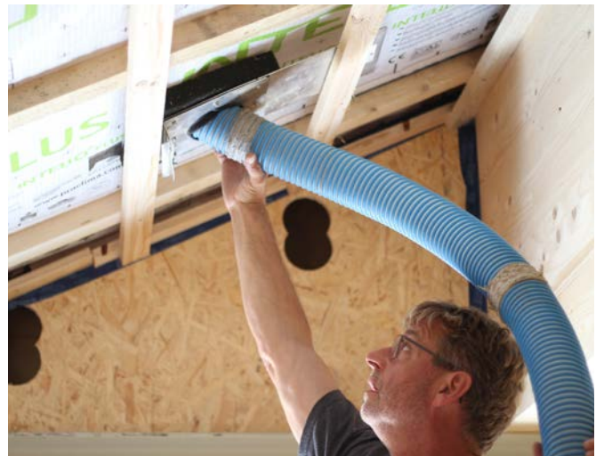
Fill roof structure using the hose procedure.
